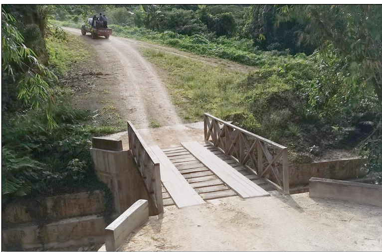
A bridge constructed by the project in Pentecost.
